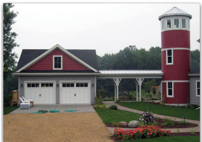
A covered walkway was added from the garage to the house.
